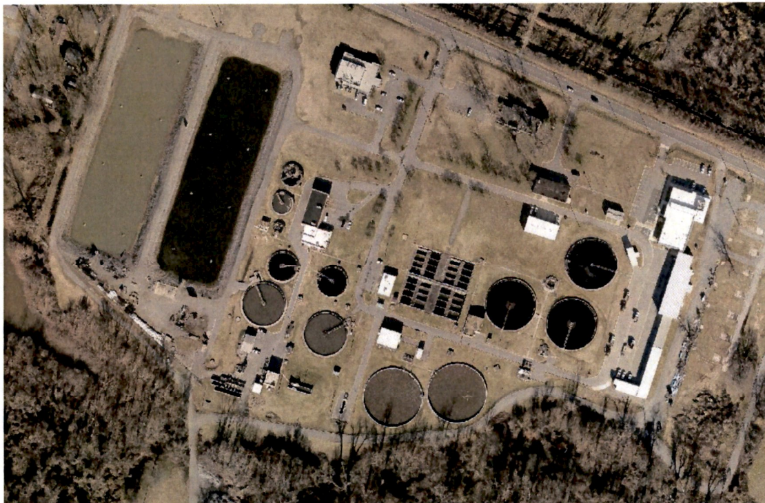
Faulkner Lake WW Treatment Plant
